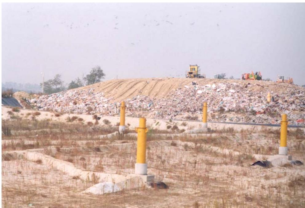
Figure 5: Gas wells for horizontal base extraction in 2001
