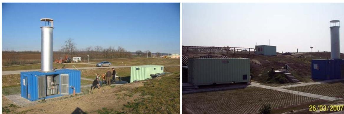
Figure 10: booster & flare, condensate shaft and manifold station in spring time 2007
